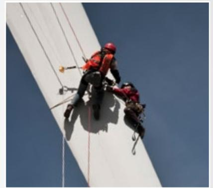
**The aerodynamic properties of the rotor blade are decisive for the performance and output of the wind energy plant. Soiling can result in turbulences and performance drops.**
